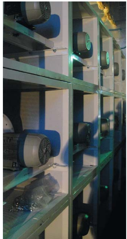
The modular design of FANWALL systems provided the ideal fan replacement solution by removing access barriers to the existing air handlers located in two mechanical rooms on the 24th floor of the CBOT building.
