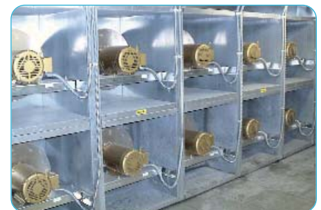
Because of its direct-drive design and smaller fan diameters, the FANWALL array has a lower acoustic impact, especially in the lower frequencies, which are more difficult to attenuate.
